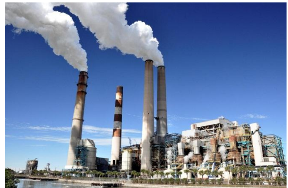
Big Bend Power Station, a coal-fired power plant in Tampa, Florida
